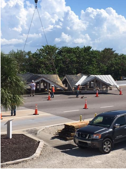
The old roof was removed and disassembled in lane three.
