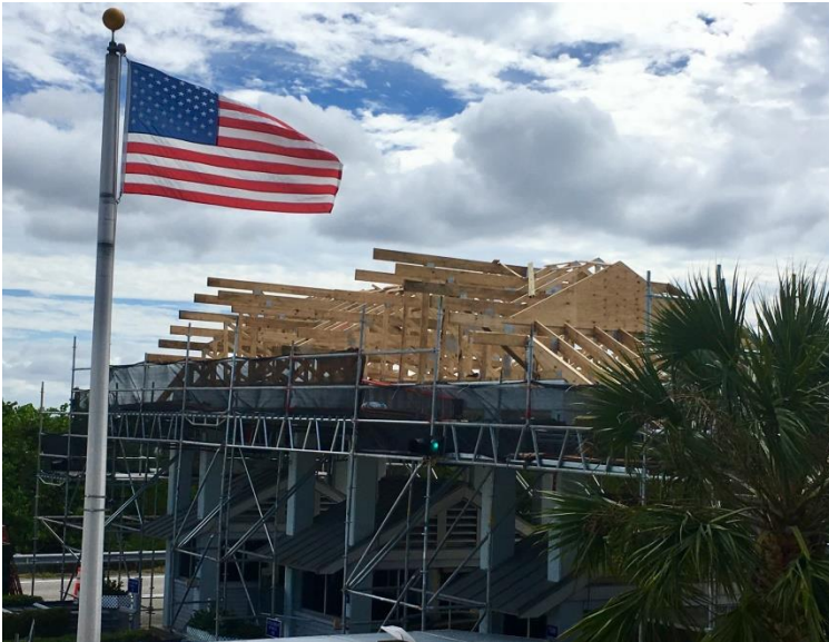
The new roof trusses being installed
